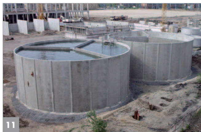
11 Precast reinforced concrete tank system for waste water treatment with fly ash concrete (XA2), (source: Benno Drössler GmbH & Co.KG/Germany)
